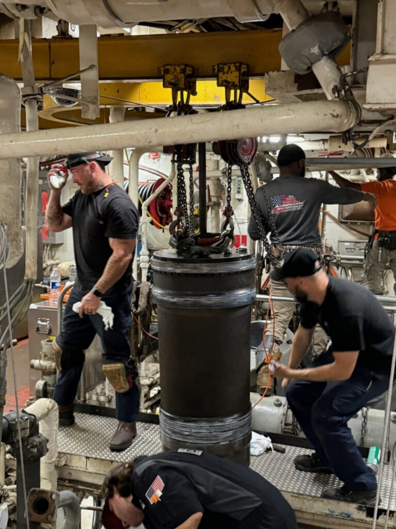
Fairbanks Morse Defense workers overhaul an engine using the
